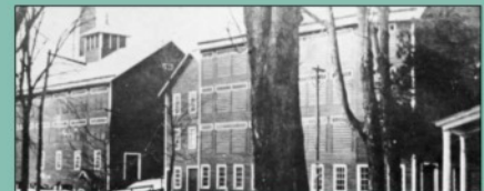
Garnar Leather Works on west side of Main Street, looking south (1910)
