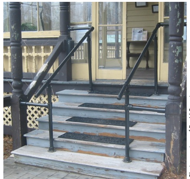
New railings on the steps of our entrance
